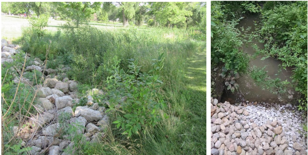
Figure 13: Rock Check Dams/Structures
