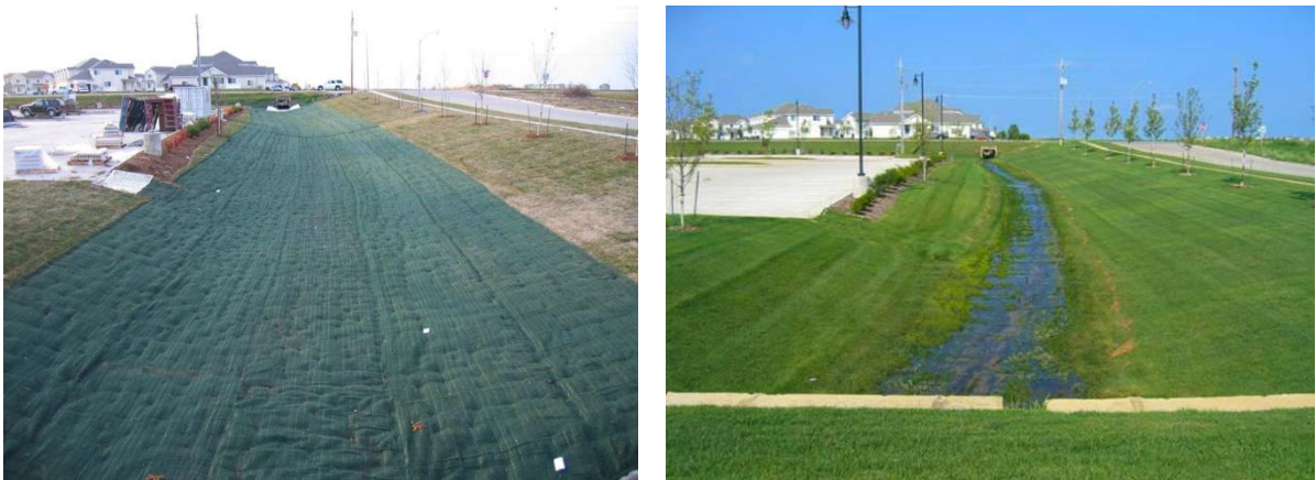
Figure 11: Turf Reinforcement Mat after Installation and Post Vegetation Establishment
