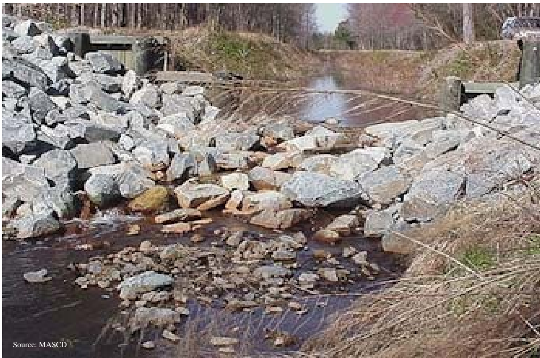
Figure 6.4.1: Rock Check Dam
