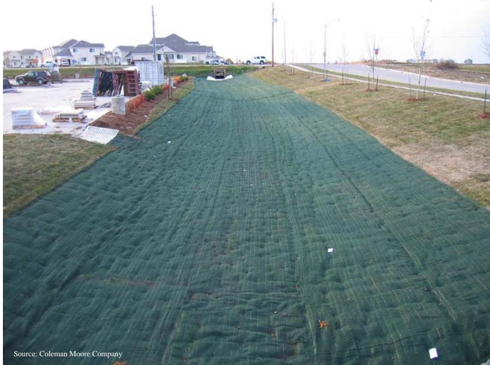
Figure 6.3.3: Turf Reinforcement Mat After Installation
