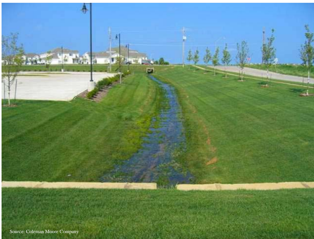
Figure 6.3.4: Turf Reinforcement Mat Post Vegetation Establishment
