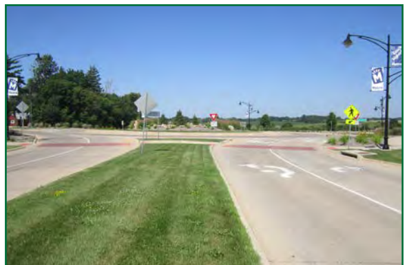
FIGURE 5: Existing Tower Terrace Road, near Alburnett Road in Marion, 2018
