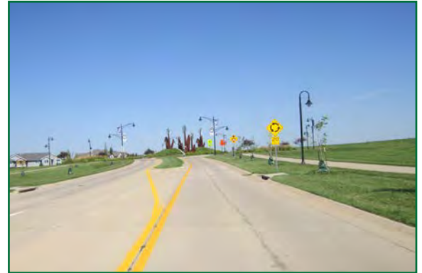
FIGURE 3: Existing Tower Terrace Road, near 35th Street in Marion, 2018
